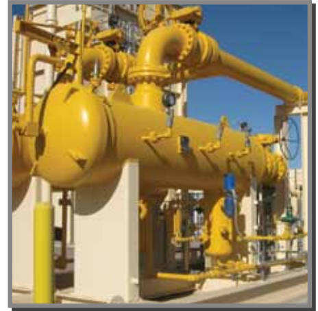
THIS ULTRA FILTER-SEPARATOR IS INSTALLED IN A METERING STATION IN CANADA. IT'S 48" HOUSING UTILIZES A FULL DIAMETER, QUICK-OPENING CLOSURE..
