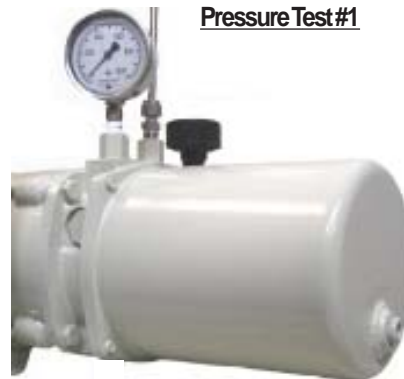
Pressure Test #1a
